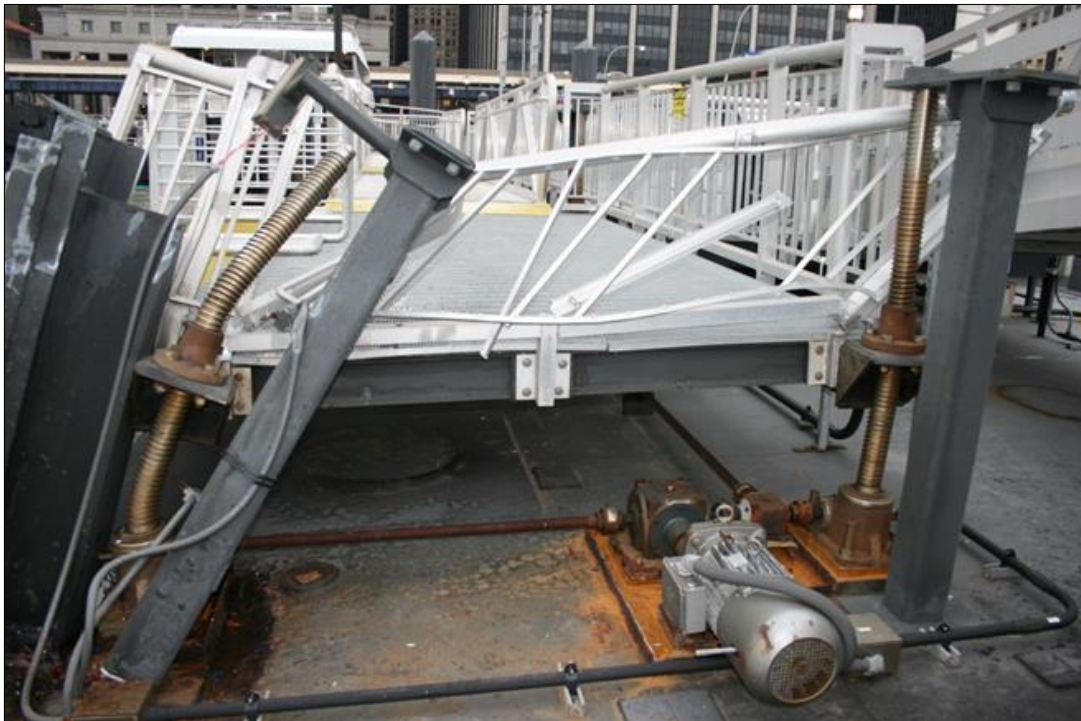
Figure 7. Damage to the Slip D2 dock barge, gangway, and upright supports.
