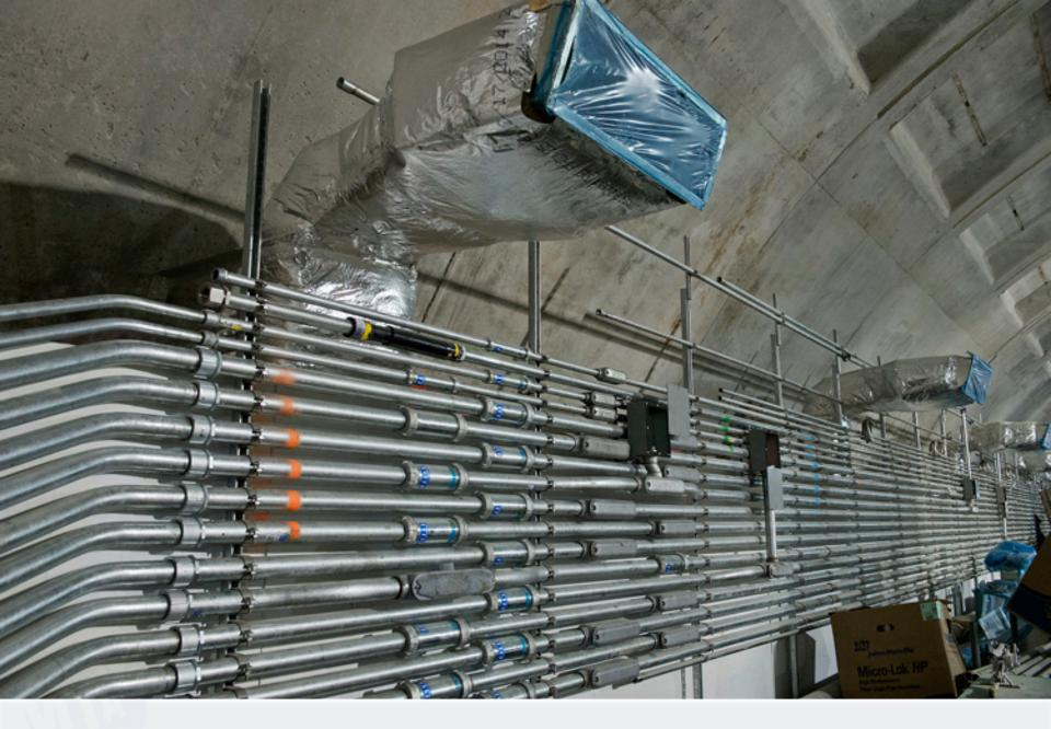
86th Street Station - HVAC duct work and conduit installation
