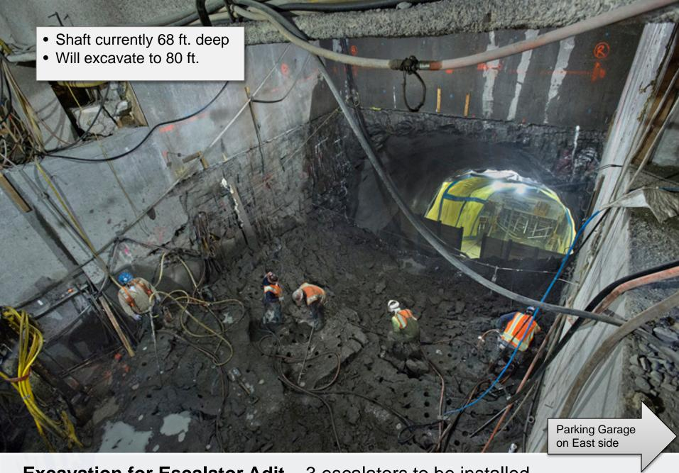
**Excavation for Escalator Adit** – 3 escalators to be installed Inside the building at 301 East 69<sup>th</sup> Street
