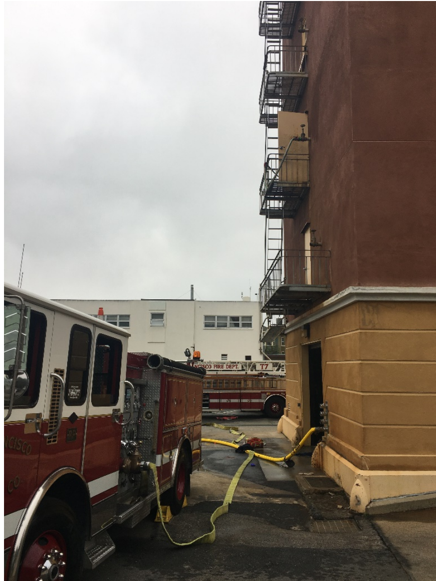
View looking East of Engine 3 and fire escape with standpipe connections
