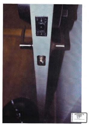
The overtorqued strikeplate caused a crack inside the doorframe. (RR10.45-46; RR17.SX26, DX40-DX41). Because the bottom of the strikeplate was driven in too far, the gap between the wood and strikeplate was exposed and the screws were torqued into the wood to the point that the strikeplate was bowed into the area where the door throw would sweep. (RR10.46).
