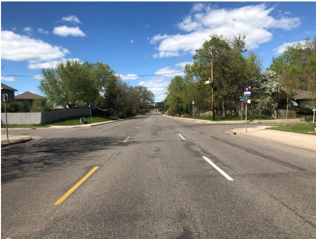
Lyndale Avenue North before with 4 traffic lanes
