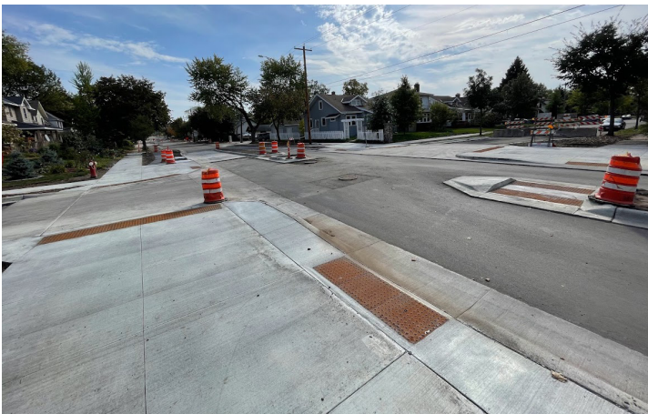
Plymouth Avenue North reconstruction
