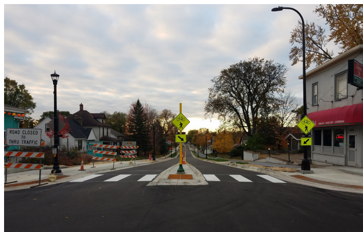
Johnson Street Northeast reconstruction
