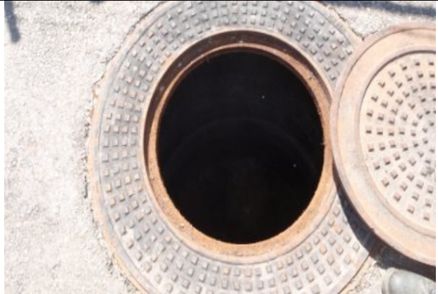
Wet well inspection at wine country lift station.
