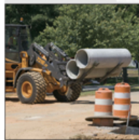
New or upgraded utilities
