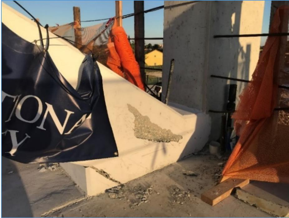
**Figure 26.** Cracks at bottom of diagonal member 11 (east view), March 15. (Source: FIGG)
