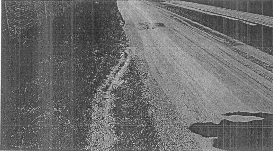
Photo 18: Asphalt strip at west edge of Eastern Service Center, this is where daily evacuation occurs of the jets on the paint striping apparatus.
