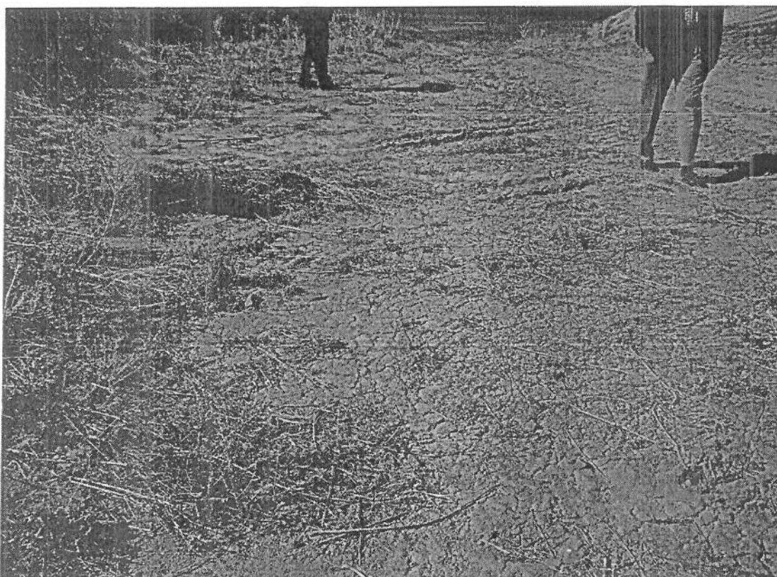
Photo 16: View of the paint dumping location looking south, note cracking of soil indicative of liquid having ponded on top of a clayey soil.
