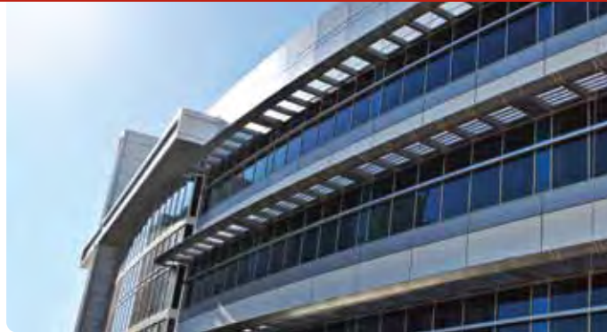
Figure 2. The new Saint John's Keck Center.
